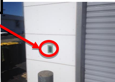
T2 Southern End adjacent to Contractor Car Park
