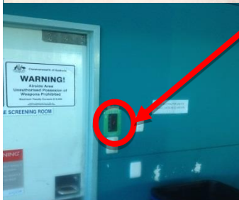
T1 Western End adjacent to check-in counter 1
